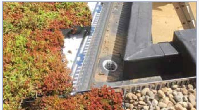
It can be mechanically fixed to the surface beneath, but if this is not possible due to the waterproofing membrane's integrity, the angle can be ballasted.
