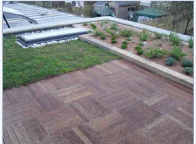
Areas such as paving or timber decking (laid onto Wallbarn ASP or TD pedestals) can be built up to the same height as the vegetation, creating one seamless garden level.
