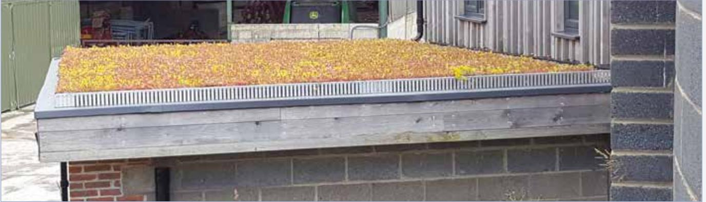
The profile is right angled, so it can sit underneath either the **M-Tray**® or the pebbles and be weighted down sufficiently.
