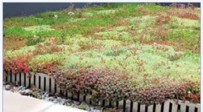
Where there is an exposed edge with no parapet, the perforated aluminium angle can be used to provide an edge to the green roof itself. It is recommended that the angle is mechanically fixed to the deck in some way. The pebbles are then installed the other side. This ensures free flow of drainage water.
